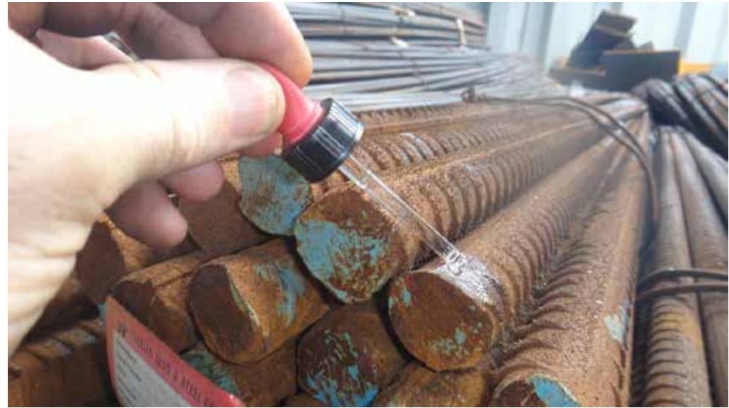
Chloride testing– steel rebar
