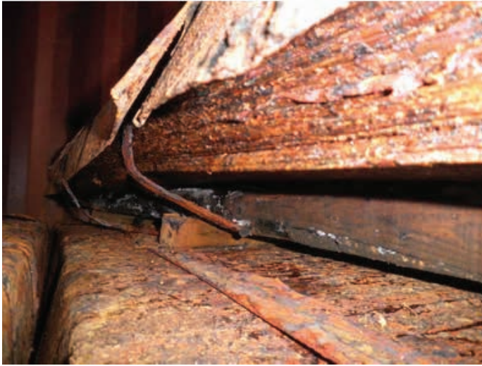
Figure 1.7 | Heavily rusted steel slabs.
