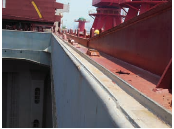
Figure 2.2 | Water drainage channel, compression bar and the landing pads as shown in good condition.
