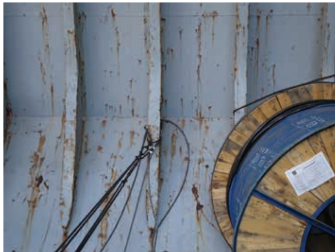
Figure 5.33 | Attaching lashings to the vessel’s side frames as seen here should be avoided.
