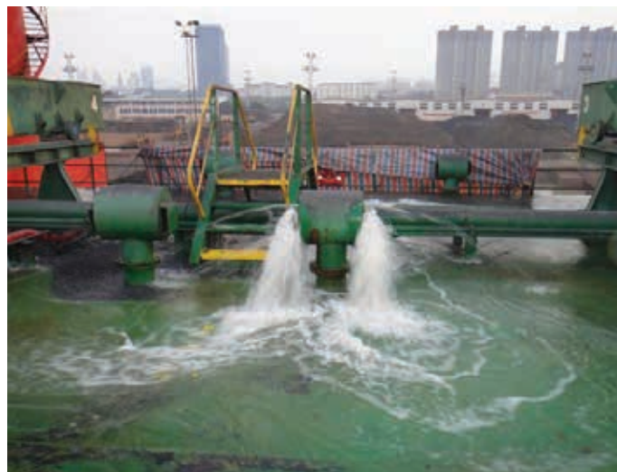
Figure 2.8 | Ballast tank hydro-testing.
