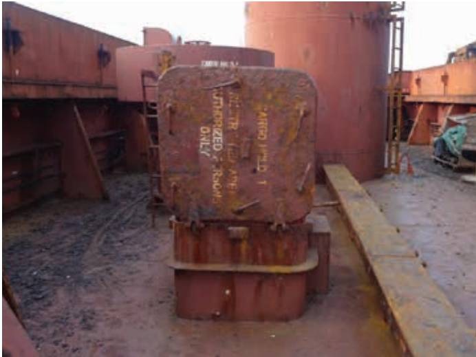
Figure 2.11 | Cargo hold access hatch in poor condition.
