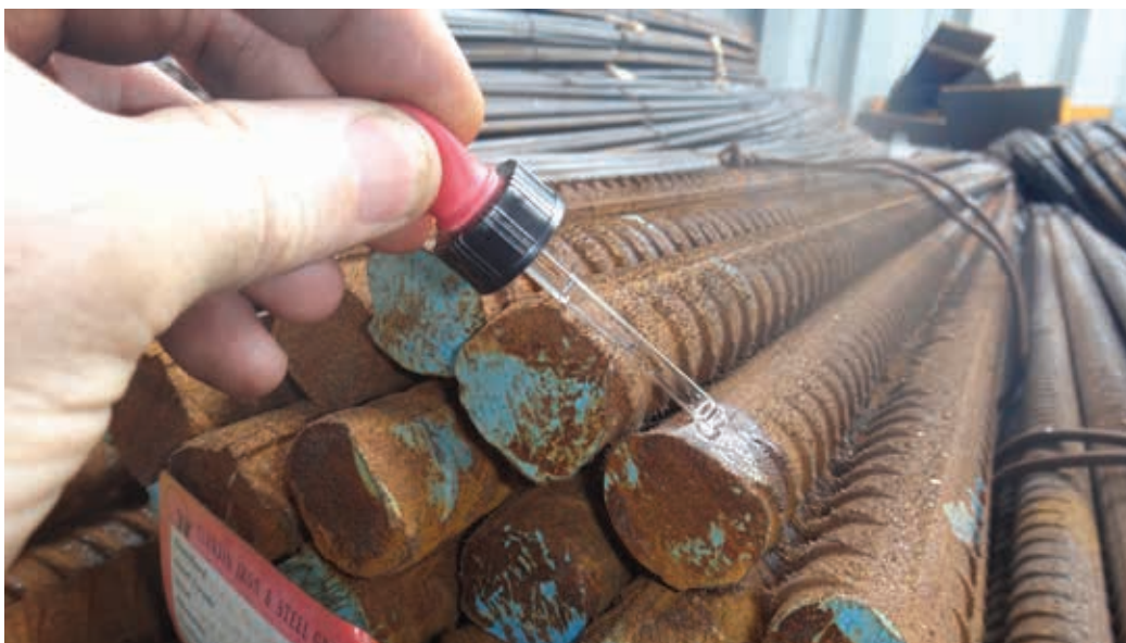
Figure 8.1 | Silver nitrate testing of steel rebar bundled with steel wire.
