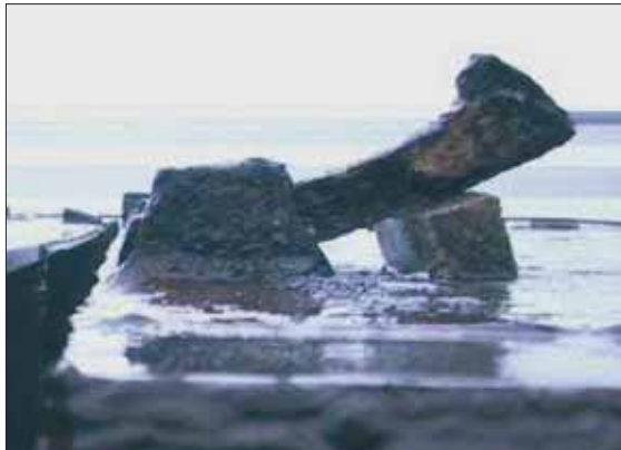
"Banana" shaped cross joint wedge
