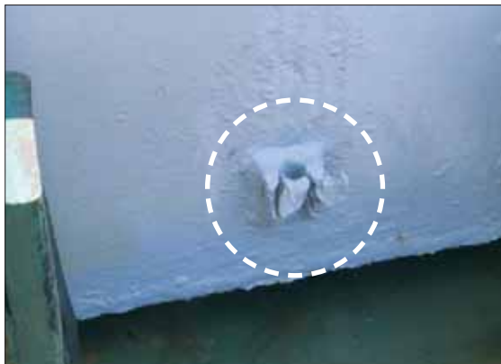
Damaged quick acting cleat snug on panel side plating
