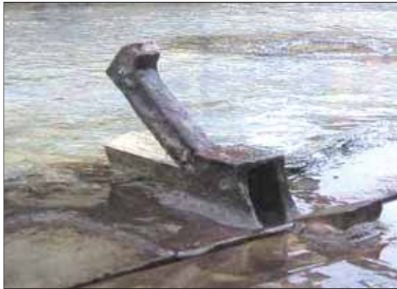
Note shipboard made triangular striker plate for cross joint wedge (bad practice)
