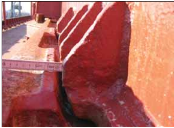
Measuring clearance in way of side stoppers
