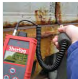
Detecting leaks with "pin-point" accuracy
