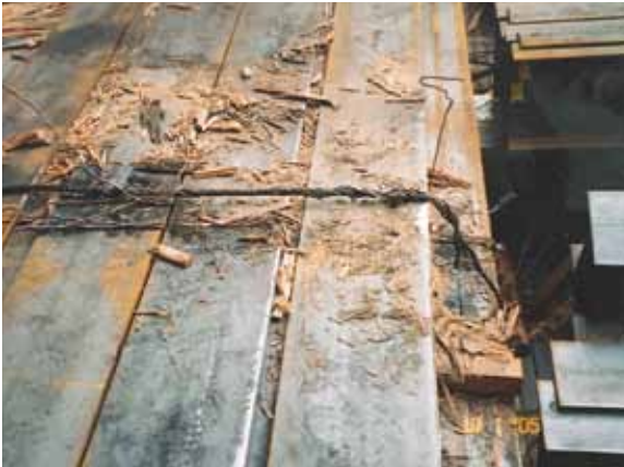
Figure 2: The timber dunnage fitted between tiers of steel products has been mangled to matchwood.
