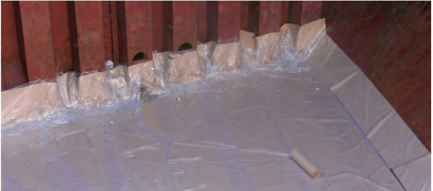
Figure 3.5 | The cargo hold top tank, base of the transverse corrugated bulkhead and base of the hopper tank top have been lined with kraft paper overlaid with clear plastic sheeting.
