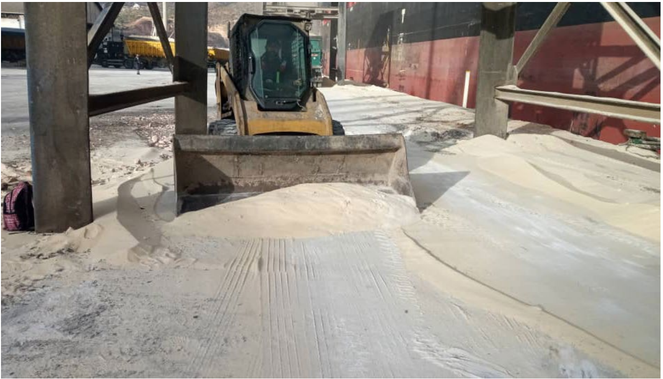
Figure 8 | Bulldozer cleaning up residual grain cargo quayside (c/o Budd Algiers)
