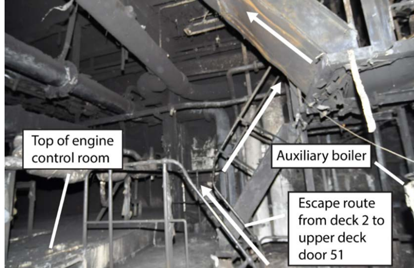
Indication of the complex route to egress in the engine room.
