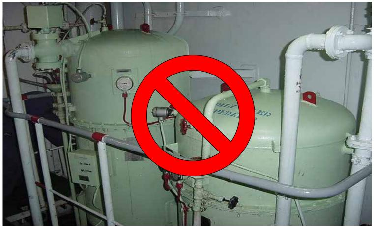
Bypass lines previously fitted; removed and pipes patched
