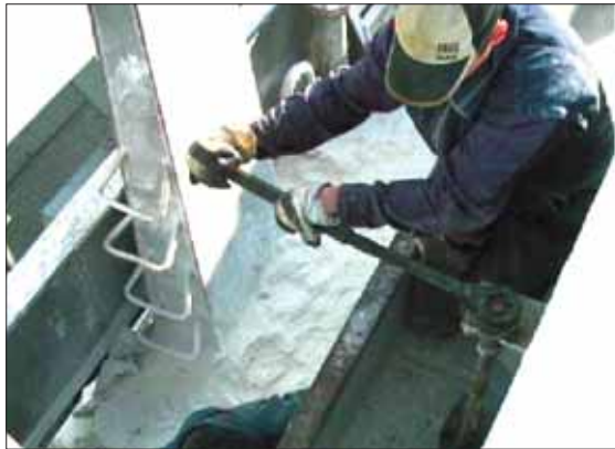
Tightening cleats with spanner and extension pipe (“cheater”)
