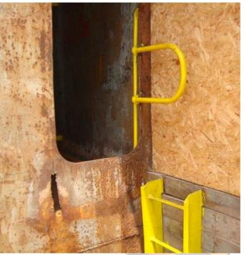
ladderwell hold design and configuration did not provide sufficient hand holds at the top of the ladder to prevent his falling. Eventually, modifications were made in order to ensure that grip bars above the ladder were installed above the ladder as seen in the figure.
